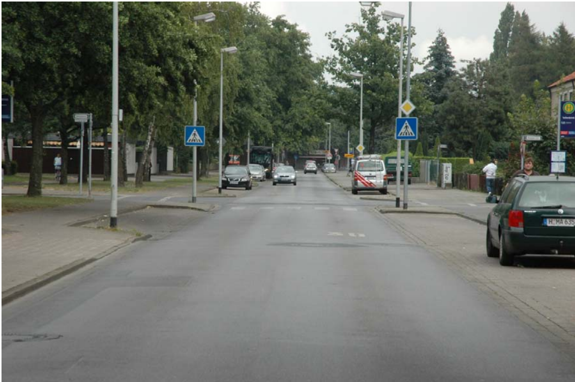
Figure 3: Eberlingstraße (installation location)
