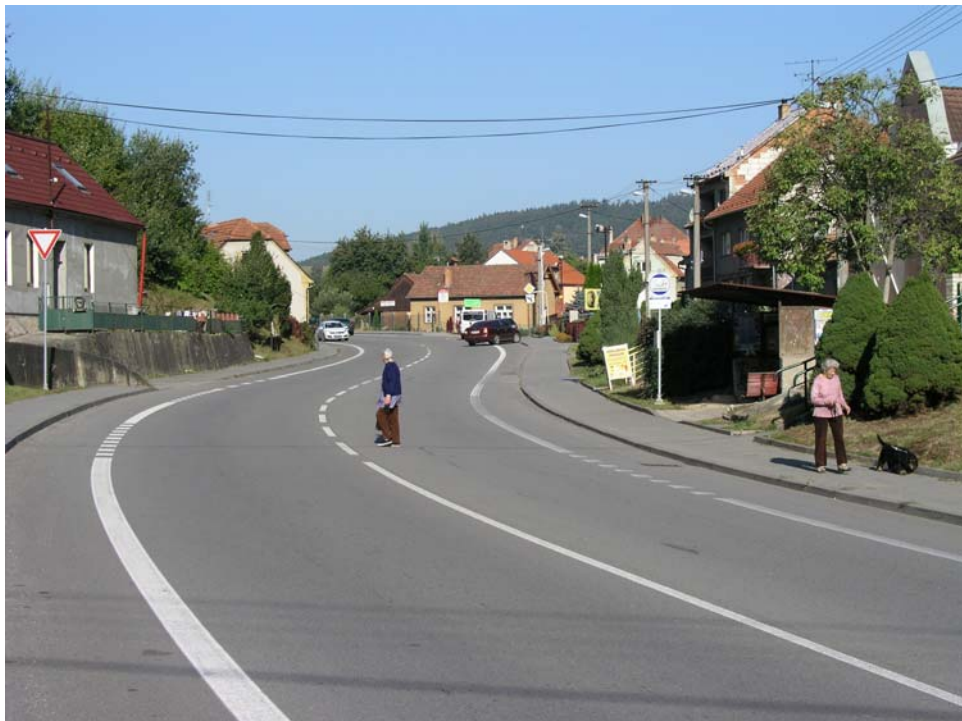
The bus stop in Šebrov – standing bus creates queues, sometimes even with illegal overtaking. There is also pedestrian crossing missing – people are used to cross the road even without it.
