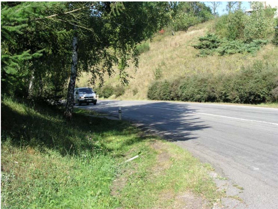
Entering the intersection in Svatá Kateřina – the priority sign is hidden in the vegetation. The sight is also not sufficient.
