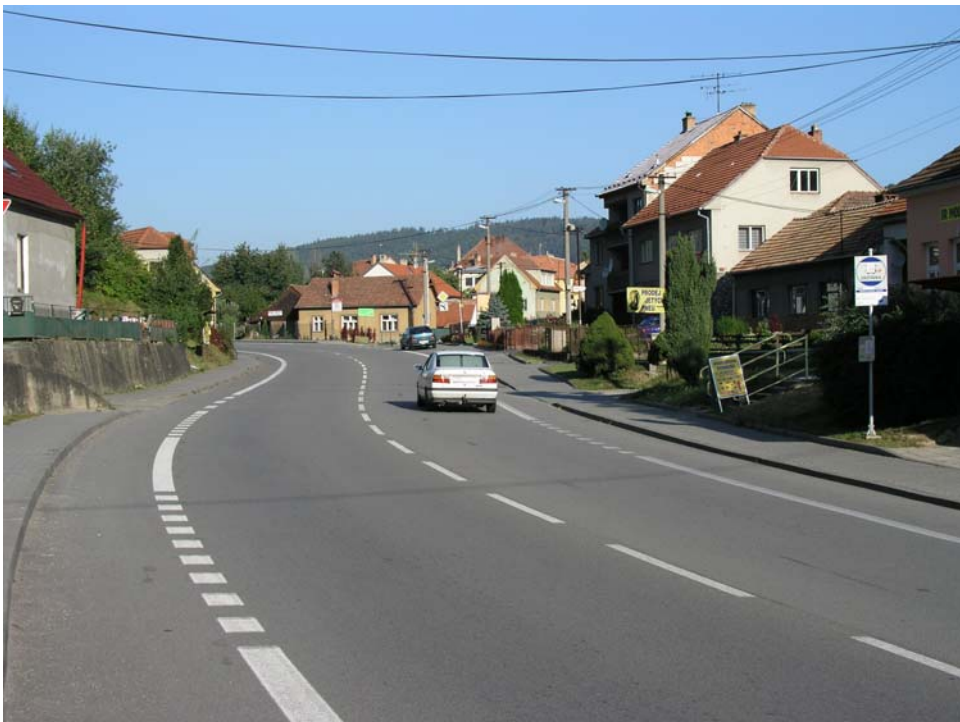
Šebrov – excessive comfort in the road width. Nevertheless, shoulders are not wide enough either for cycle lane or parking lane.
