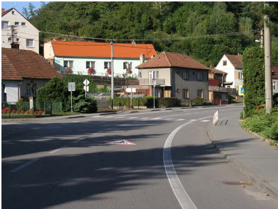
Pedestrian crossing in front of elementary school with insufficient road signing and marking – both the warning sign on the right and the symbol on the ground are hardly visible.
