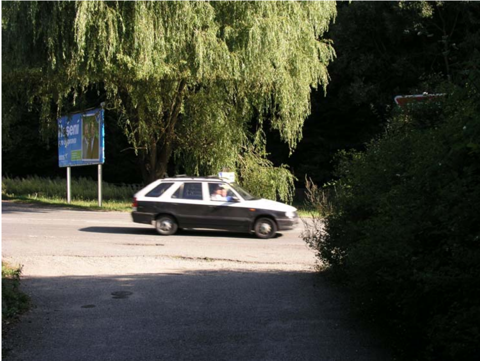
Entering the intersection in Svatá Kateřina – the priority sign is hidden in the vegetation. The sight is also not sufficient.
