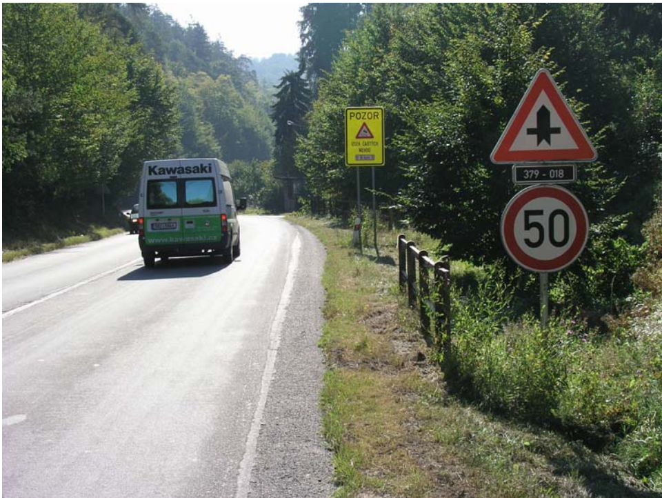
Road signs indicate the risk and order to slow down without any evident reason – the road is not self-explaining.
